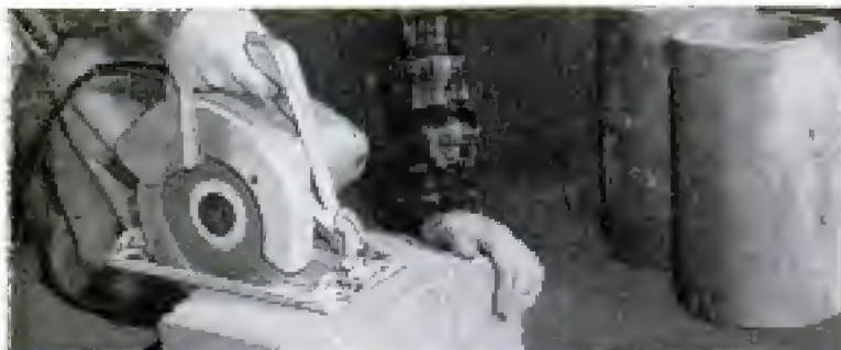
Above, note similarity of operations of cutting wood and clay tile. Saw is held in same manner. Woodcutting blade is replaced by abrasive disk for cutting tile. Right and below, saw squares up broken pieces of hollow tile and concrete for re-use
